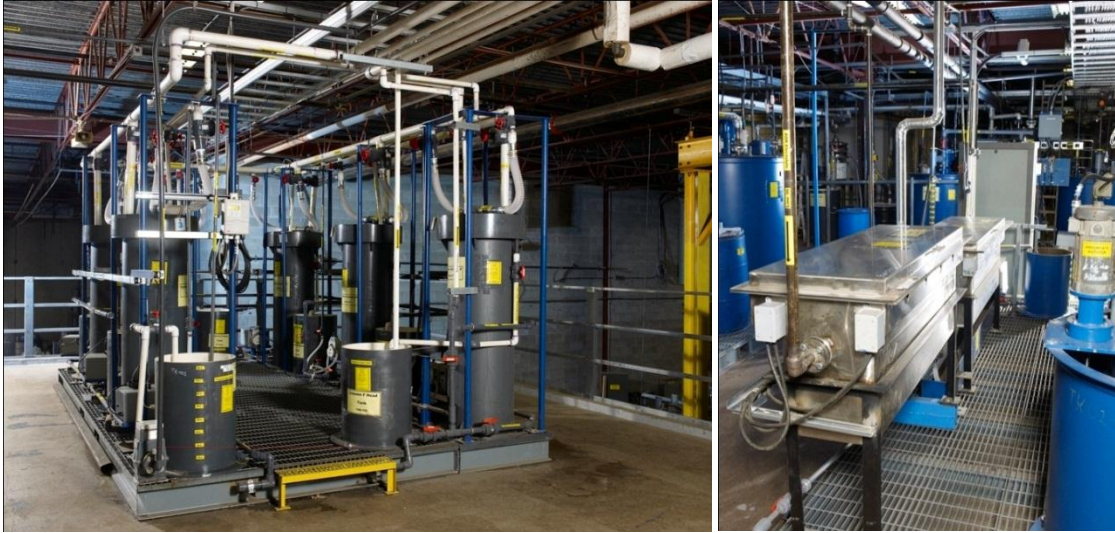
Figure 5 - CESL Gold Demonstration Plant ADR Circuit (CIC and EW Cells)
